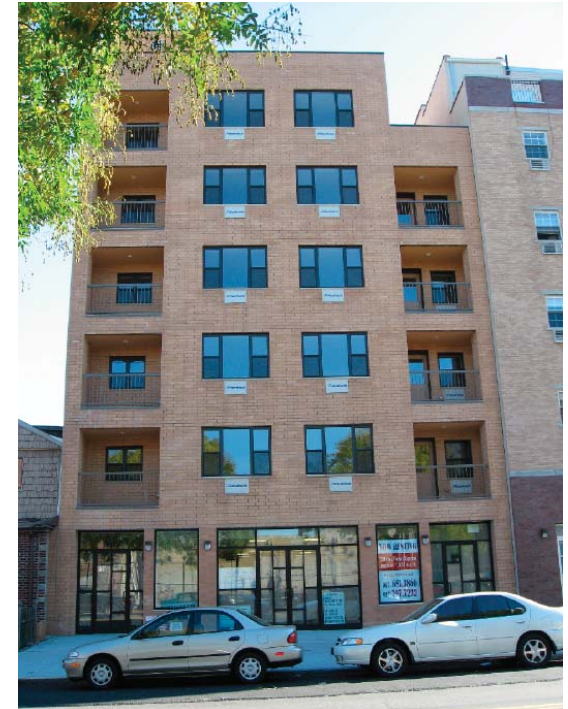
New residential construction: this example on a small infill lot on Second Avenue signifies the area's strong housing market.
