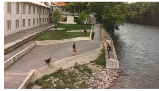
This project utilizes a historic riverfront mill site to mitigate flood inundation. In the sections between former canal walls (once used for the mills production efforts) wave-like terraces have been built into the terrain as a defense mechanism. Precedent: Factory by the Water River: Limmat - Zurich, Switzerland
