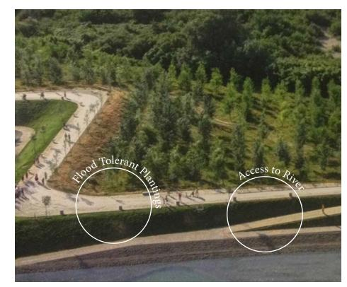
An earthen berm storm barrier serves as a bike and pedestrian route with access ramps to the lower level waterfront edge. Precedent: Parque Del Agua River: Ebro - Zaragoza, Spain Image Source: Prominki
