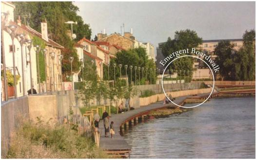
This riverside area has been divided into two levels. The existing promenade has been retrofitted with a 1meter high embankment wall that also serves as a parapet for site lighting. The second (lower level) terrace is built just above the mean water level at the water's edge. Precedent: Quai des Gondoles River: Seine - Choisy-le-Roi, France
